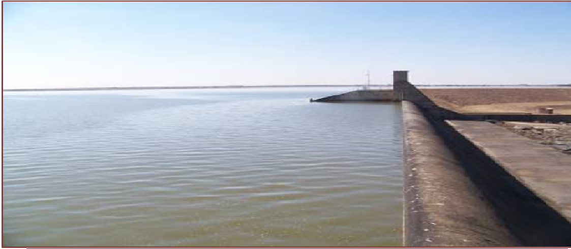
Figure 15. Water reservoir Bethlehem
