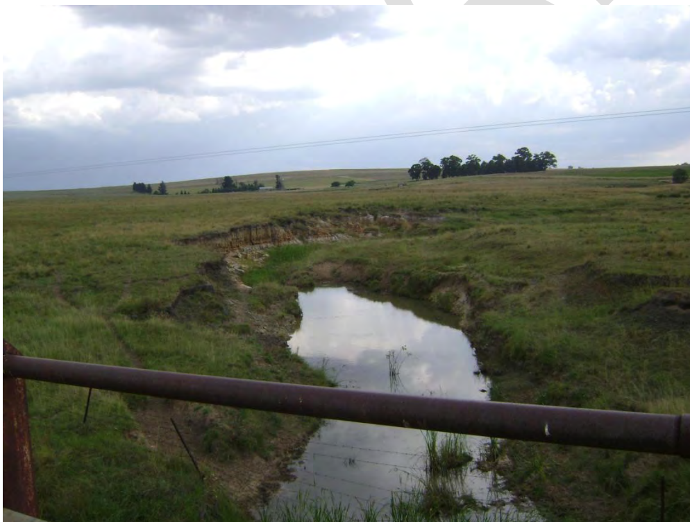
Photo 8: Lat -28.09911; long 28.45631; Description: Bridge over a stream
