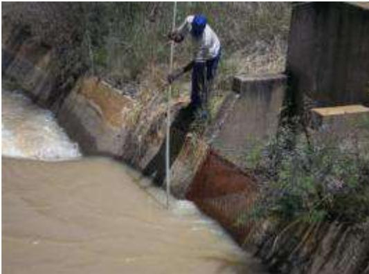
*Removal of debris from the strainer at the raw water abstraction*
