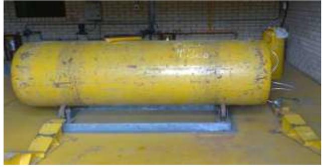
*Chlorine gas used for disinfection*
