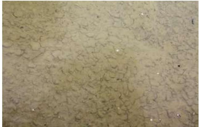
*Examples of sand filter surfaces: muddy and uneven*
