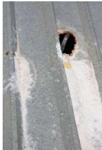
*No liquid chlorine or standby pump was available - HTH was dosed through the roof promoting further deterioration of roof*
