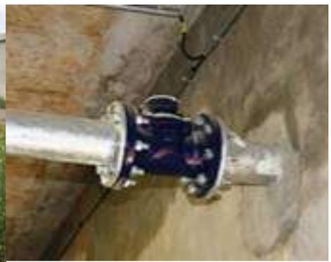
*Installed water meter close to the roof – cannot be read without ladder*
